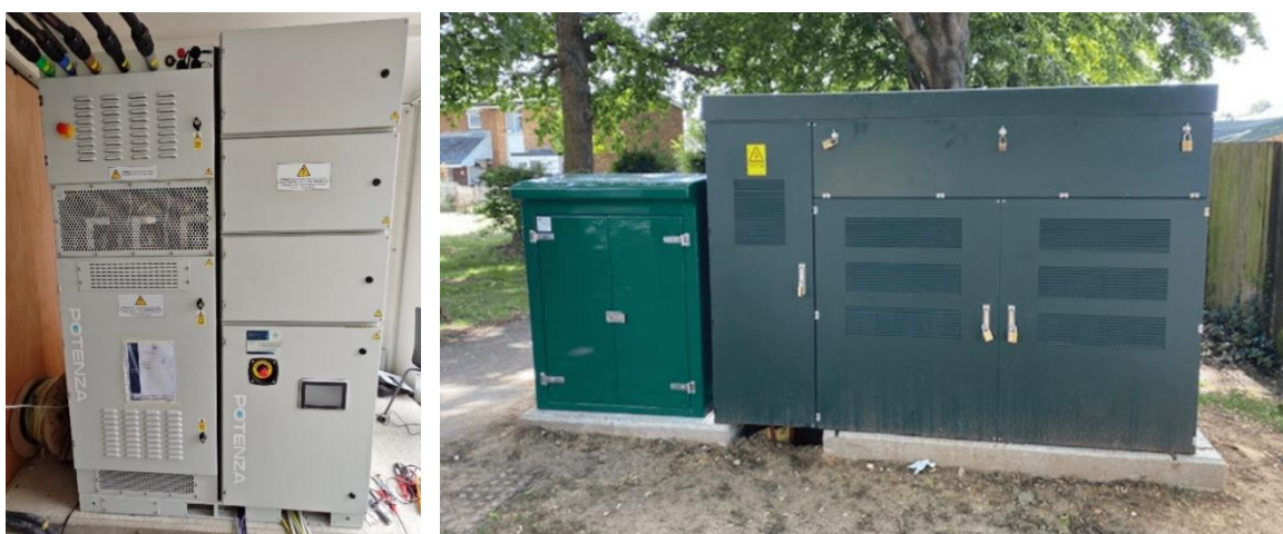
‘Potenza’ Inverters for Micro Grid EV Charger systems (Left) and Soft Open Point Grid capacity expansion (Right)
